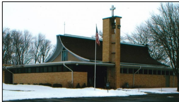
The old church was torn down and a new one was built.
